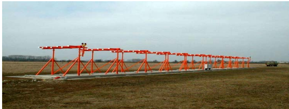
Fig. 1. The localizer antenna
