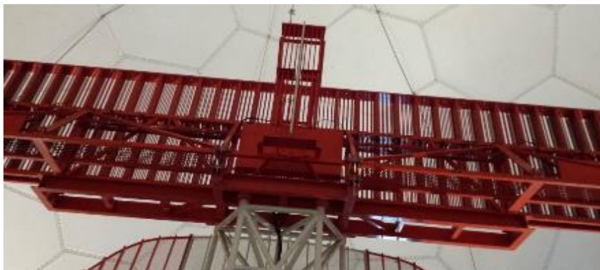
Fig.16 MSSR LVA Antenna Back Radiator [9]
